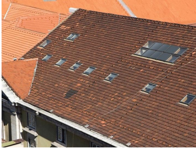
Integration STS in the roof cover
