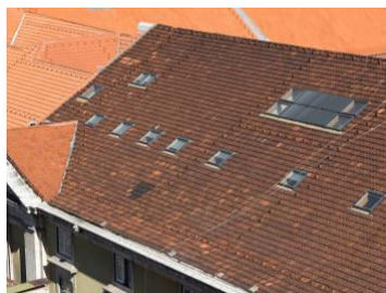
Integration of solar thermal panels in the roof cover
