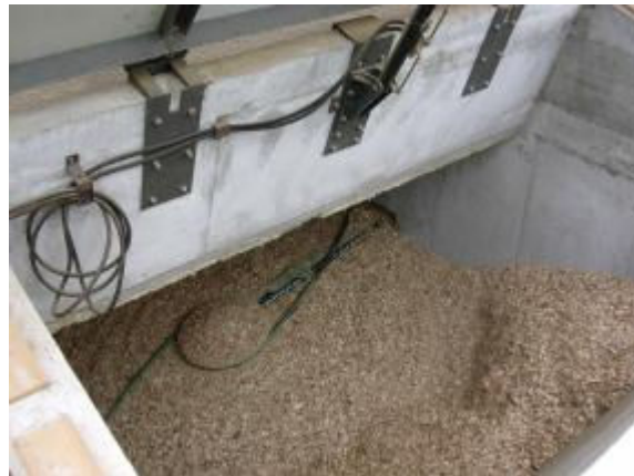
Wood chip boilers 2 MW
