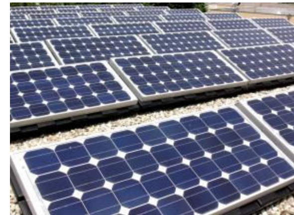
Photovoltaic systems 250 kWc
